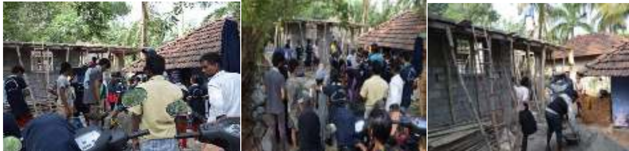
ABHAYAM-HOME FOR HOMELESS – SUNSHIDE CONCRETING
