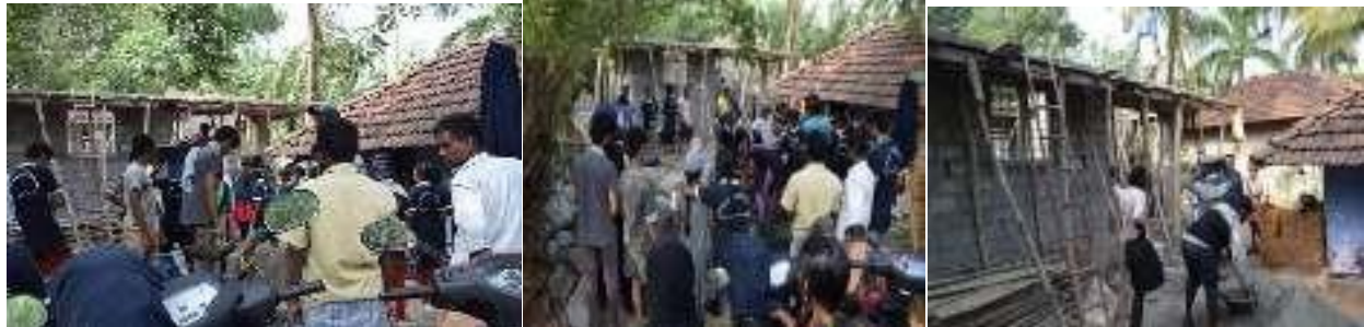
ABHAYAM-HOME FOR HOMELESS – SUNSHIDE CONCRETING
